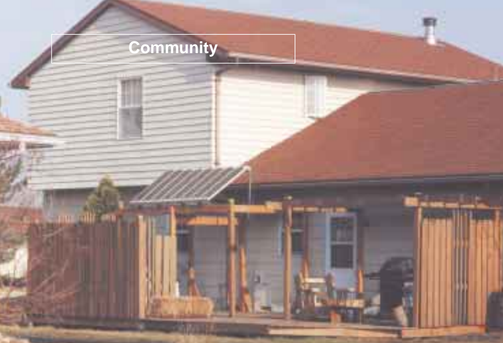
Linea Bara's home sports eight Arco Solar 16-2000 PV panels.
