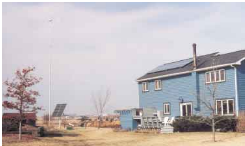
Steve and Jan Bell's system has 2,980 watts of PV and a 4 KW wind generator. See the article on page 8 for a complete description of the system.
