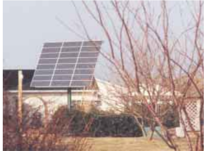
Paul and Karen Wagoner have eight roof-mounted Siemens SR-100s and twenty-four SM-55s on a tracker.
